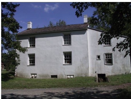
Back of Locktender's House drying out after Irene: note: basement door torn off hinges. Photo: C. Leedom
